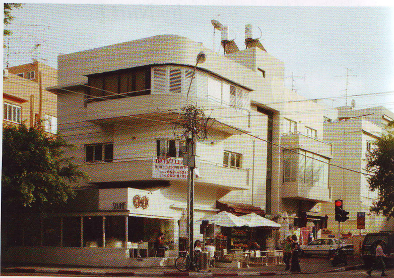
A typical Bauhaus-inspired building on Frishman Street 2008
